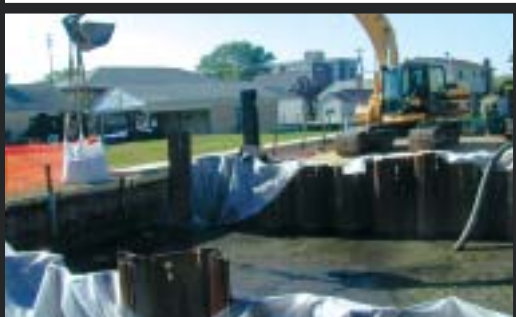
Sorbond is used to solidify contaminated soils or sludges that can ultimately be disposed of in regulated waste facilities.
